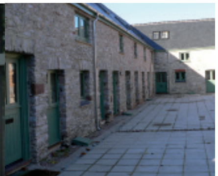
Gerald Wood Homes (Midas) Architect: Heighway Field Associates Project Location: Berry Pomeroy
